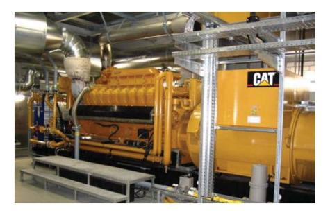
10 x G3520C's used for Municipal District Heating with Detachable Water Module Over 89 % Thermal Efficiency
